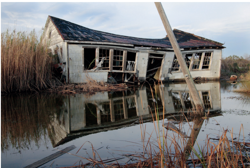
A house destroyed and lifted off its foundation by Hurricane Katrina, in Irish Bayou, New Orleans, LA. © iStockphoto.com/Chad Purser
